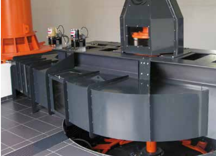
AUSTRIA Theuerwangwehr power plant Kaplan pit turbine 408 kW
