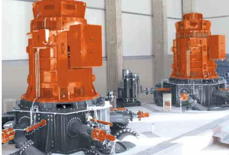
ARMENIA Vardenik power plant Pelton turbine, 6 nozzles 2 x 3270 kW
